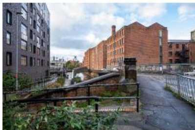
View C: Existing View
