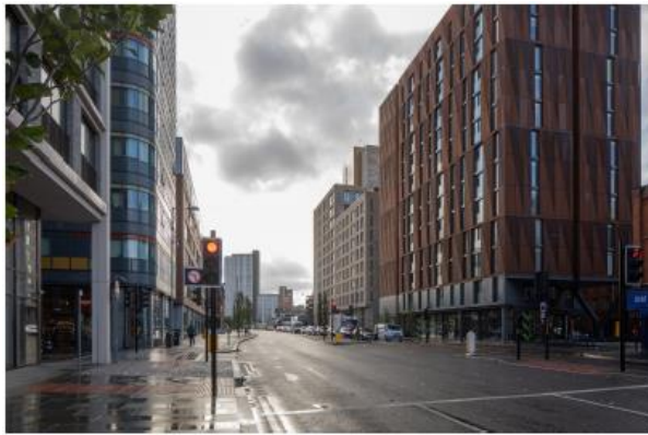
View B: Existing View
